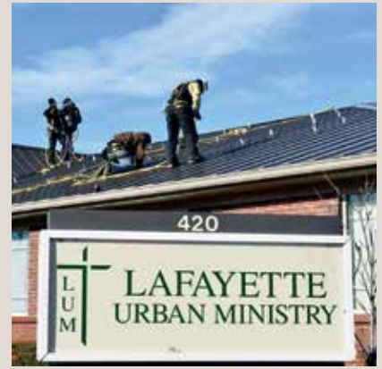
New roof and solar panels help power LUM programs.
